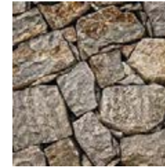
To Retaining Walls + Sign Wall
